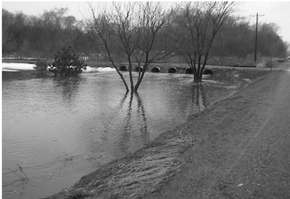
Figure 3.10: High flow through culverts under a side road, February 25, 2000.
