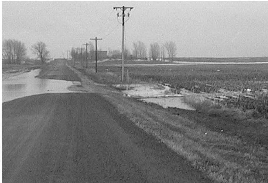
Figure 3.11: Ponded melt water flows over the road, February 25, 2000.
