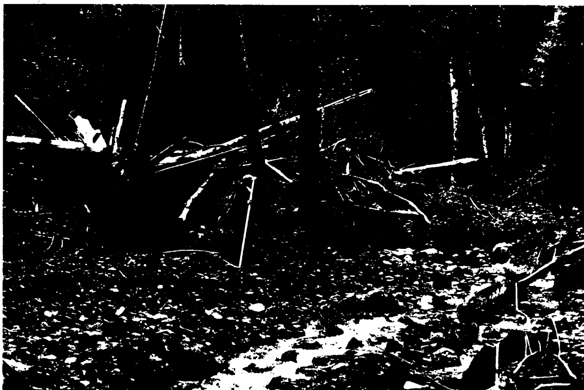
Fig. 4.5 Upstream view of stalled organic dam on Huckleberry Creek (location shown in Figure 4.4, approximate elevation 300 m).
